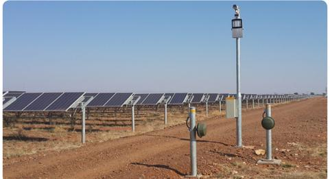
The client's requirement was for a single operating platform with a map display interface that would allow for real time monitoring of all CCTV camera analytic alarms, all microwave barriers and all alarm systems. The system also needed to control 36 LED light fittings on the perimeter that were to be used as "surprise lights" that would light up when the microwave barriers were triggered.
