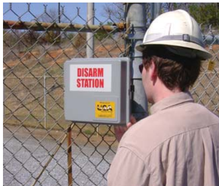
A disarming system allows entry for utility personnel and approved contractors, but keeps copper thieves out.
